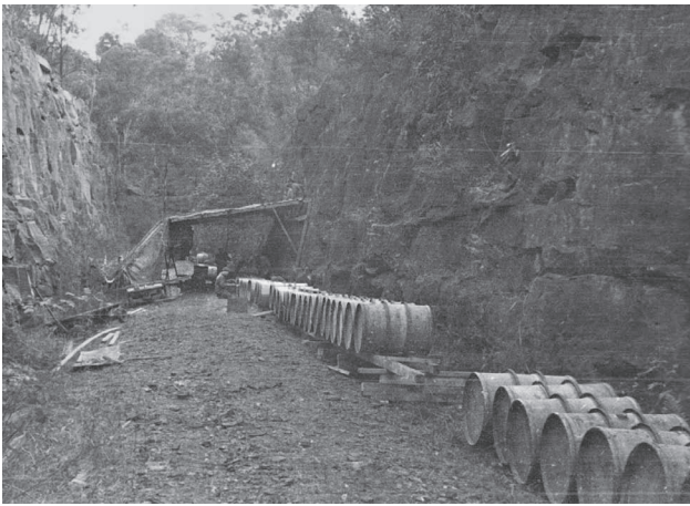
East cutting to chemical warfare storage tunnel at Glenbrook where the maintenance of the bulk storage containers was undertaken. To the right mustard gas drums are seen in bond (a settling period after venting) and other drums are being cleaned and repainted by a chemical warfare armourer under a tarpaulin which spans the cutting. Mid-1943.
